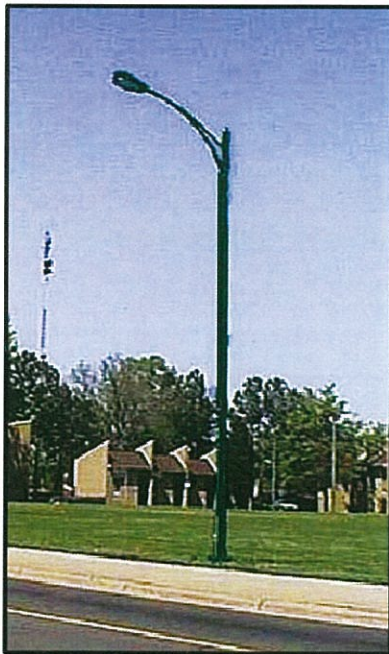
GREEN PAINTED STEEL POLE
