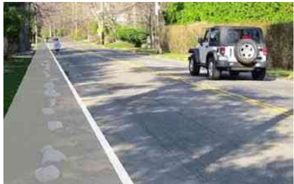
widened and striped, with rocks moved
