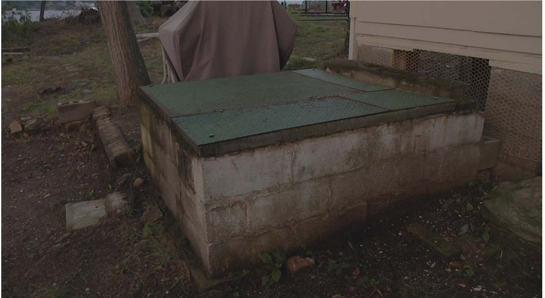
Above ground sewage pit
