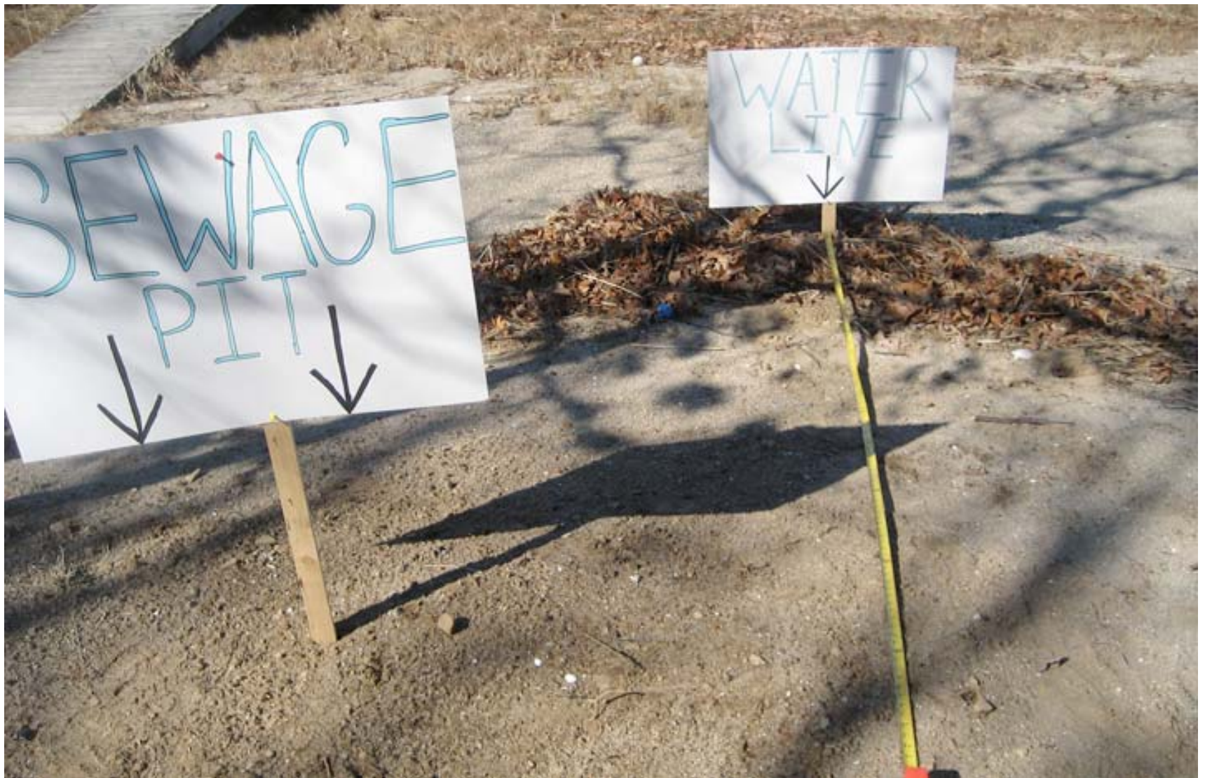
Sewage Pit, 7 ft. from high tide water line
