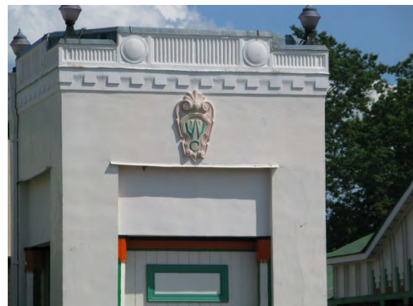
Playland's mix of uses and Art Deco details make it very distinctive.
