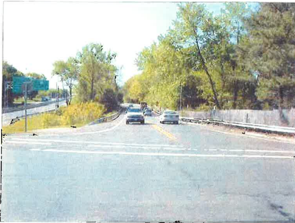
PLAYLAND PARKWAY NORTHBOUND ON/OFF RAMP AT OLD POST ROAD, LOOKING NORTH
