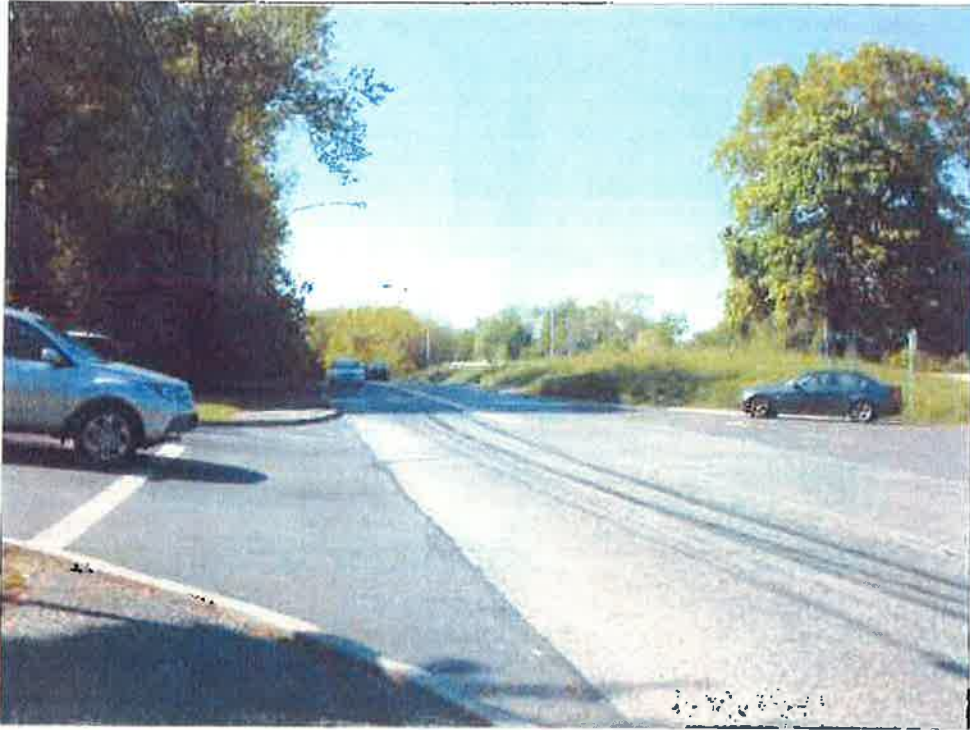
PLAYLAND ACCESS DRIVE AT MEDICAL OFFICE ACCESS DRIVE/ PLAYLAND PARKWAY SOUTHBOUND ON/OFF-RAMPS, LOOKING NORTH
