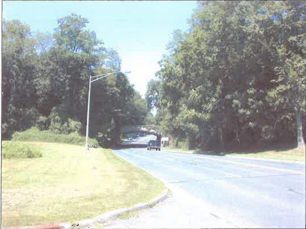
Playland Parkway at Ramp from U.S. Route 1 Looking West
