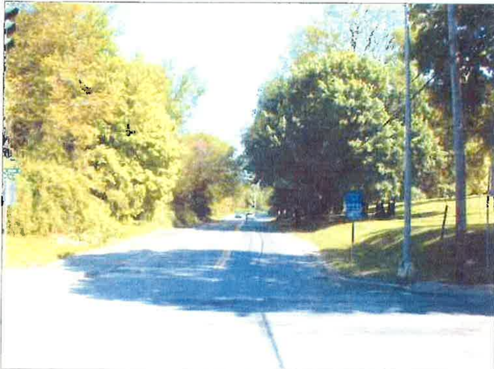
PLAYLAND ACCESS DRIVE AT THEODORE FREMD AVENUE, LOOKING SOUTH
