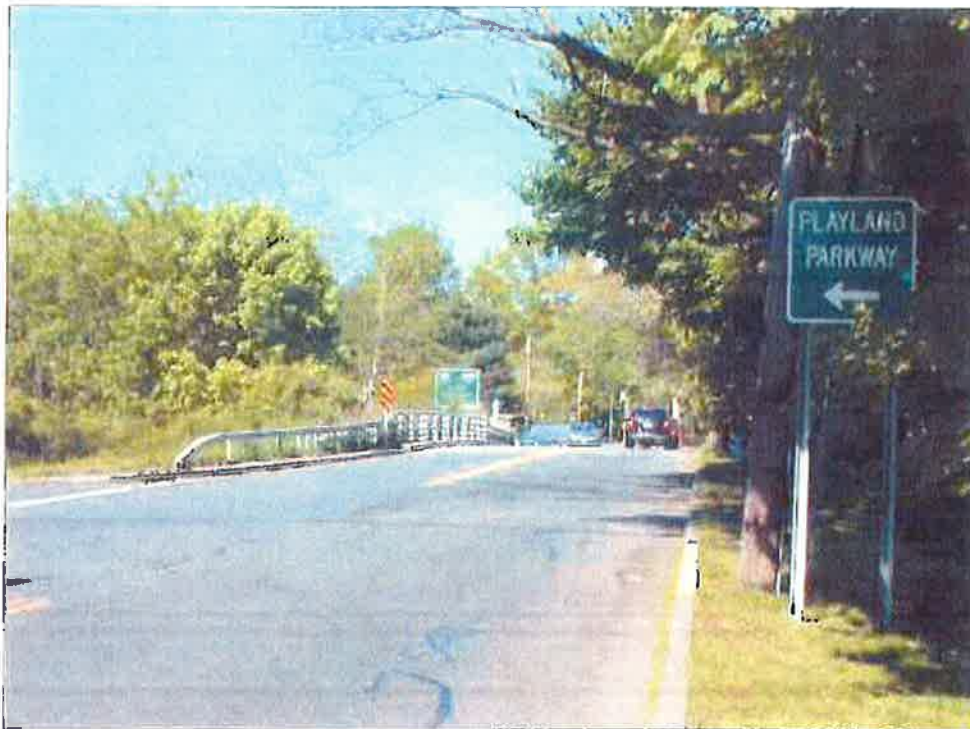
OLD POST ROAD AT PLAYLAND ACCESS DRIVE, LOOKING EAST
