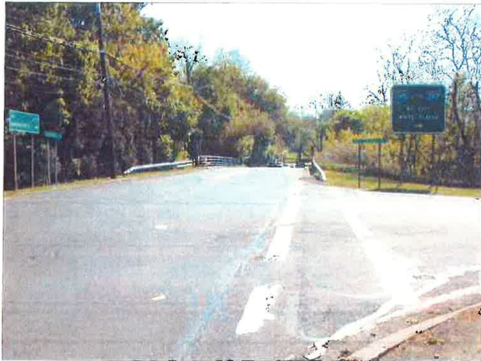
OLD POST ROAD AT PLAYLAND PARKWAY NORTHBOUND ON/OFF RAMPS, LOOKING WEST
