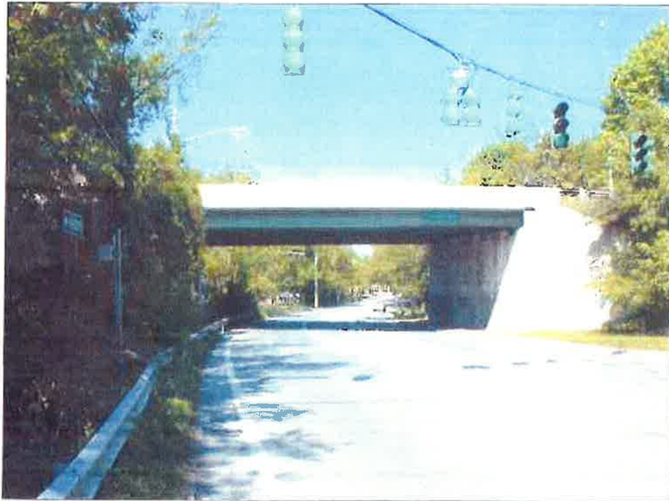
THEODORE FREMD AVENUE AT PLAYLAND ACCESS DRIVE, LOOKING EAST
