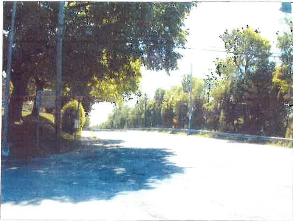
THEODORE FREMD AVENUE AT PLAYLAND ACCESS DRIVE, LOOKING WEST
