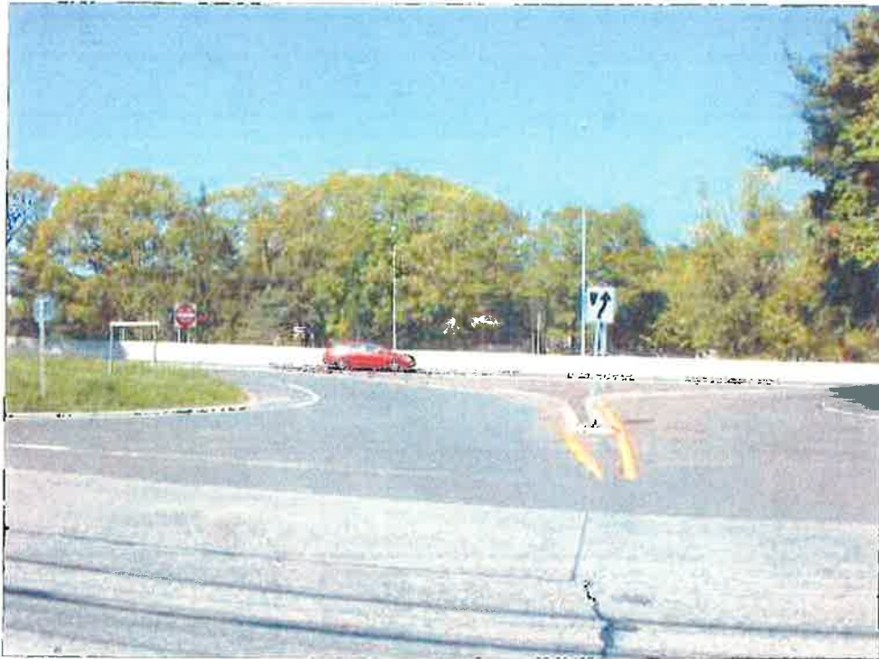
PLAYLAND PARKWAY SOUTHBOUND ON/OFF-RAMP AT PLAYLAND ACCESS DRIVE, LOOKING EAST
