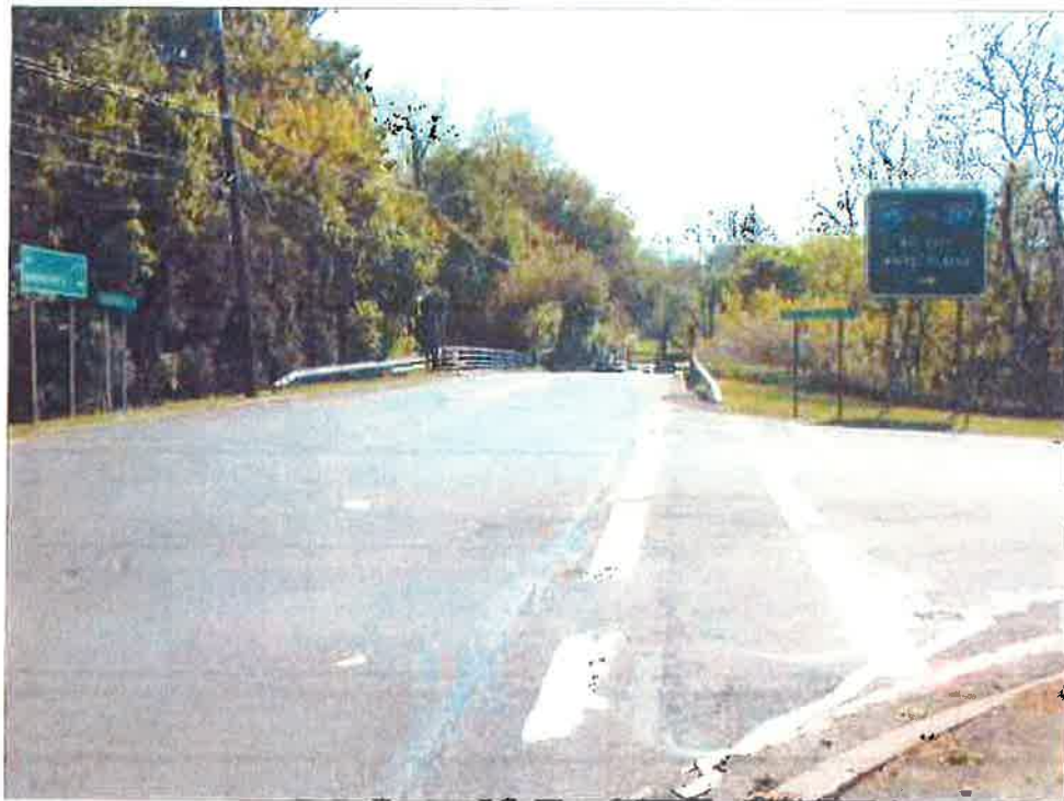
OLD POST ROAD AT PLAYLAND PARKWAY NORTHBOUND ON/OFF RAMP, LOOKING WEST
