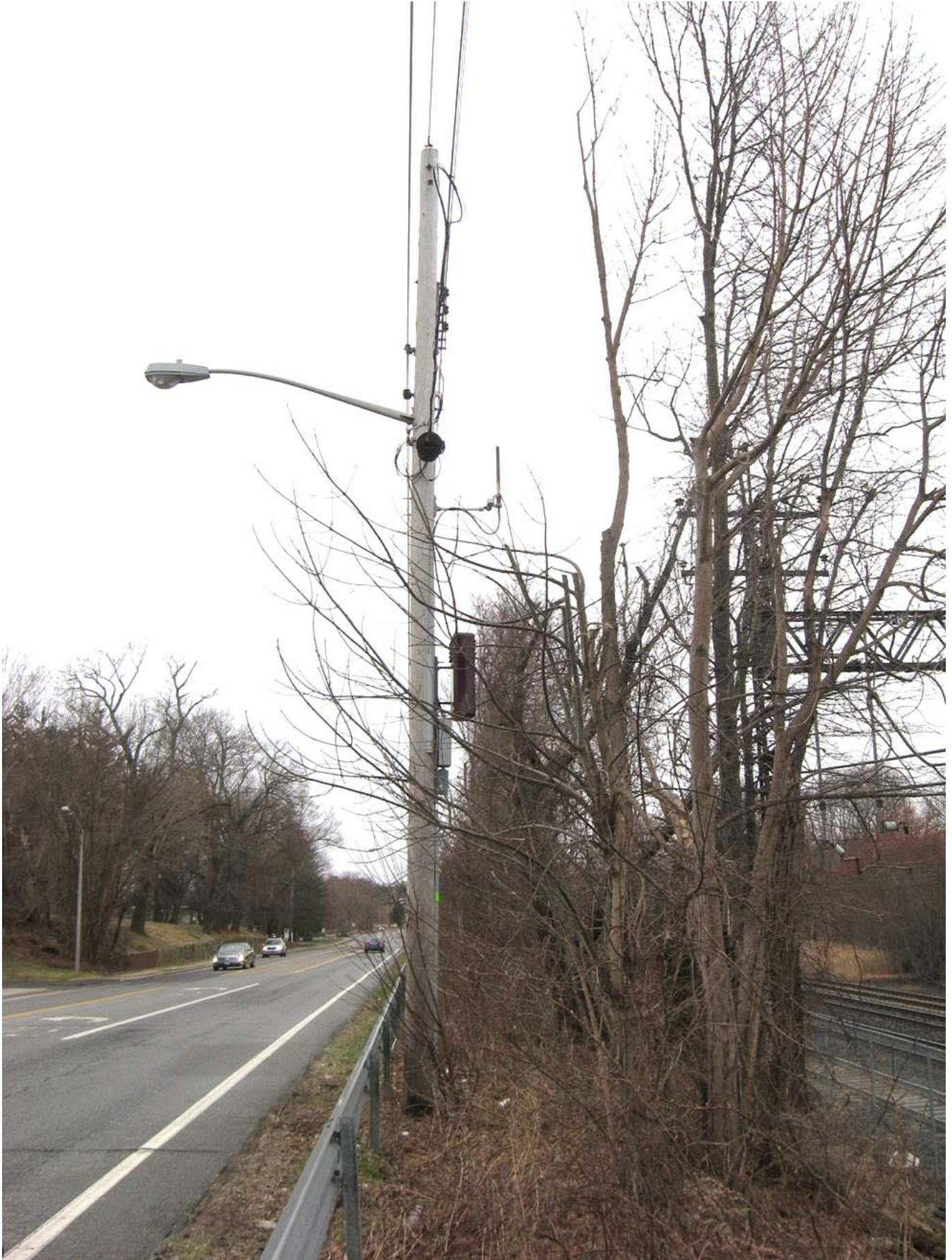
NYD6387 Comm Zone Installation - Across from 401 Theodore Fremd Ave
