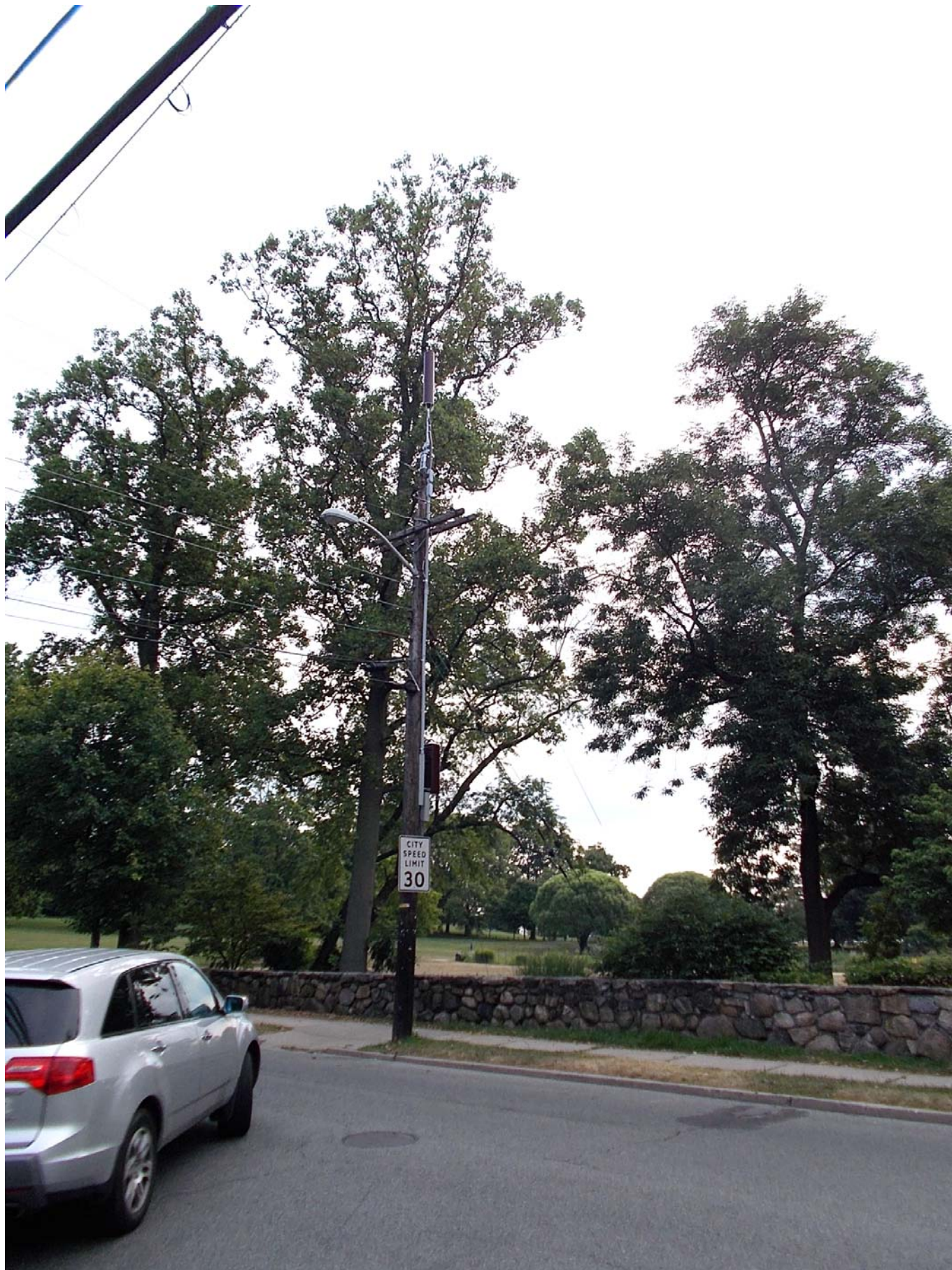
NYD6382 Pole Top Installation - Across from 594 Forest Ave
