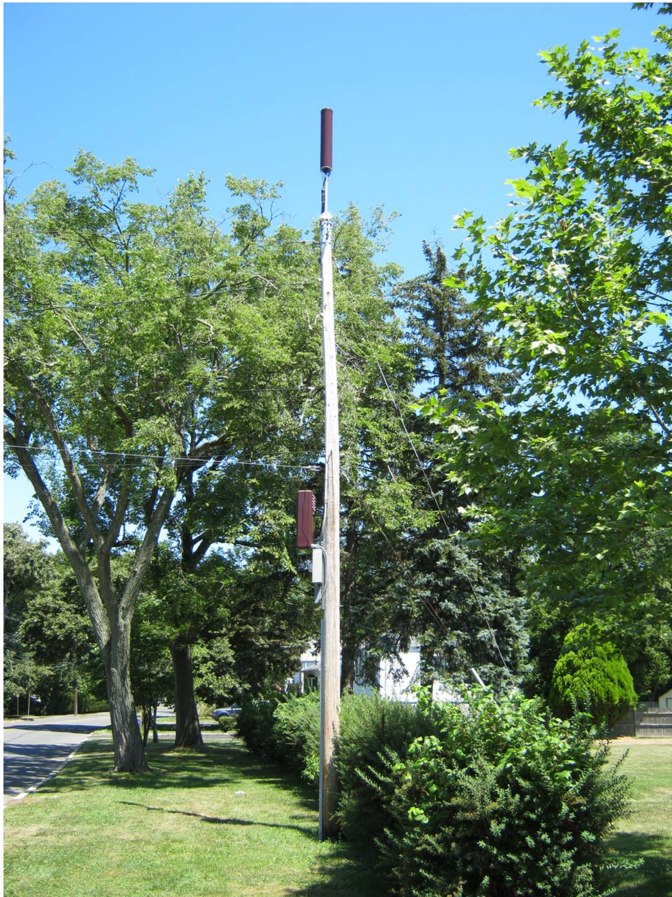
NYD6383 Pole Top Installation - Side of 411 Milton Rd (50ft South)
