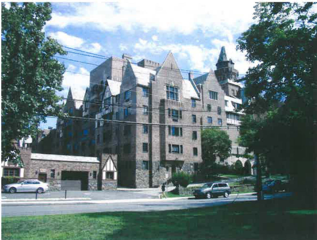
West Elevation Photo 1 of 2 – North End
