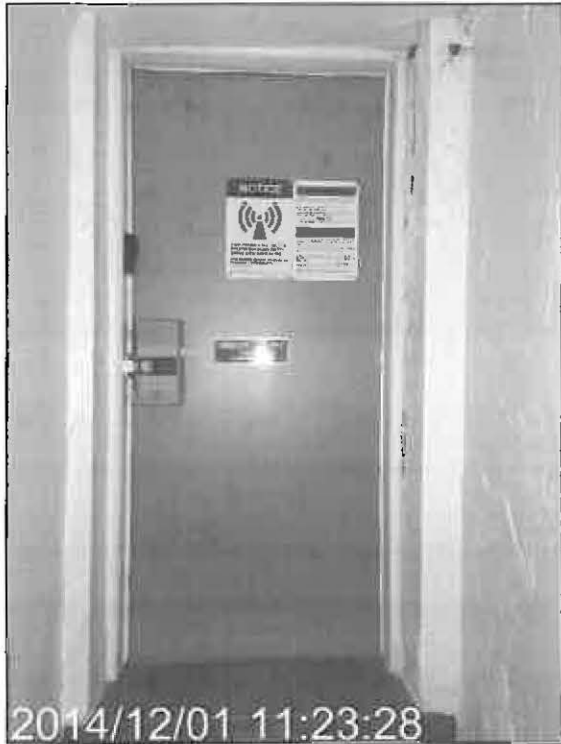
Access 1 – Existing Notice Sign, Guidelines sign required
