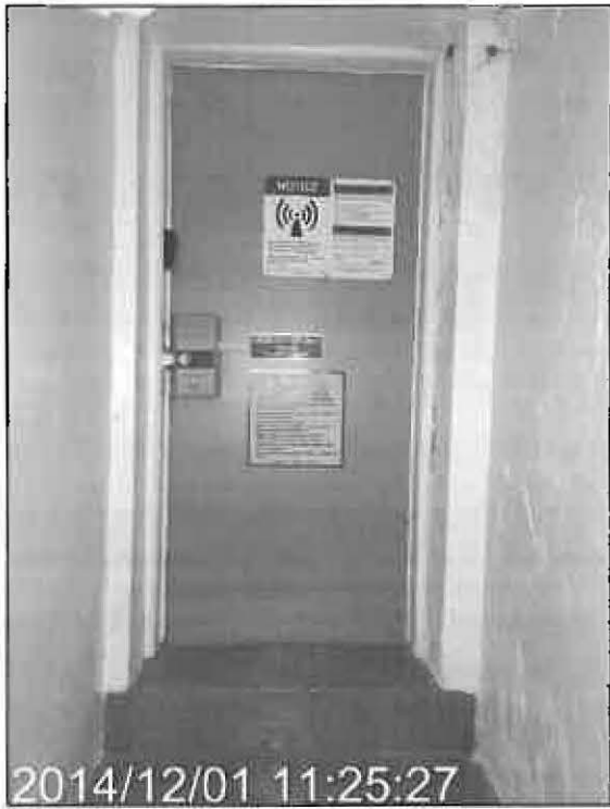
Access 1 – Existing Notice Sign, Guidelines sign Posted
