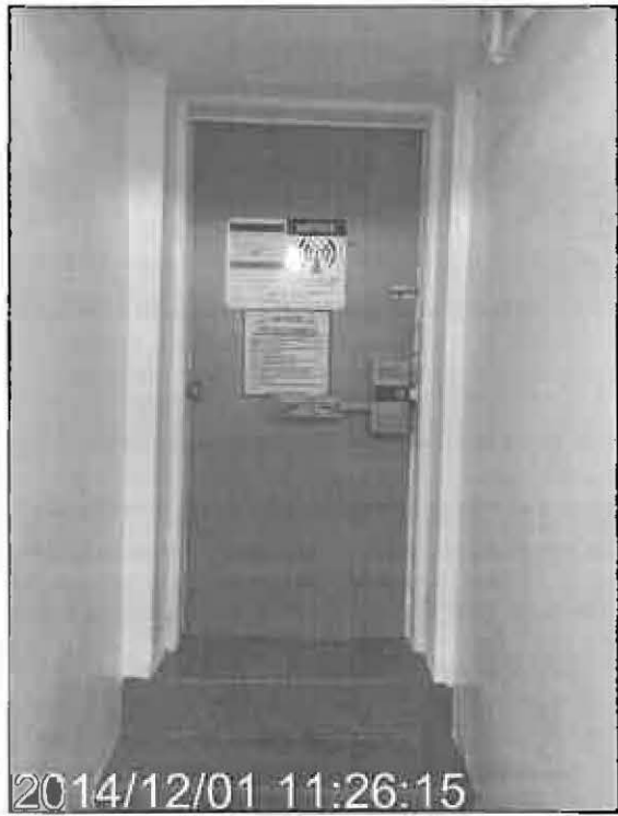
Access 2 – Existing Notice Sign, Guidelines sign Posted
